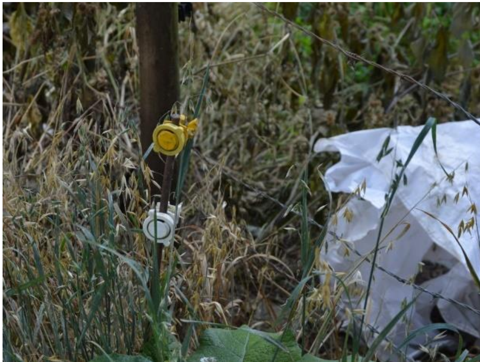
Electric fencing had once been installed but was currently non-operational
