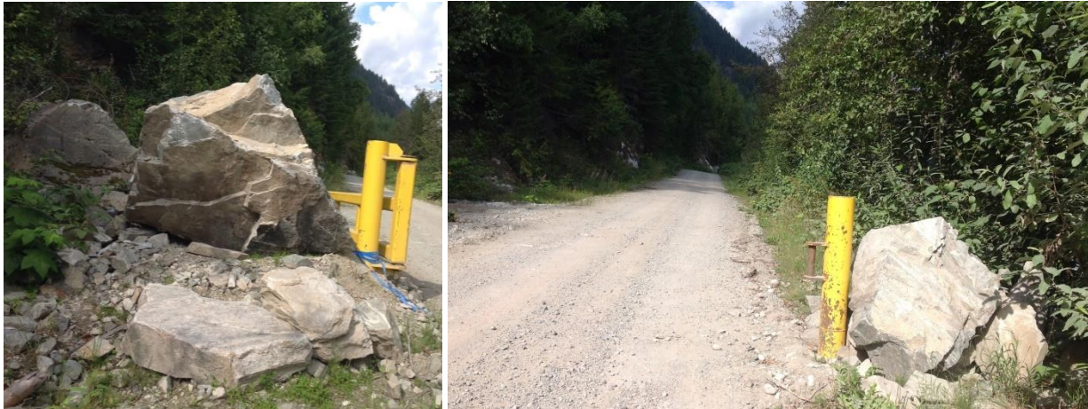
During closure the boulders on either side of the gate discourage people with motorized vehicles from going around the gate.
